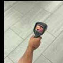
Check floorheating for leaks
