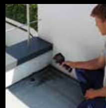
Discover leaks in roofs
